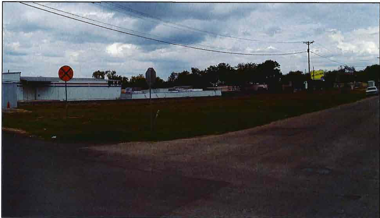
Subject property facing north from Katy Street.
